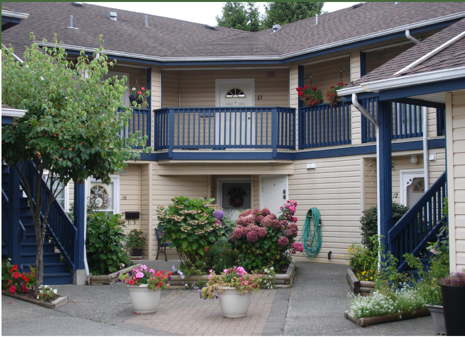
Blueberry Vale Housing Co-operative, Richmond, B.C.
