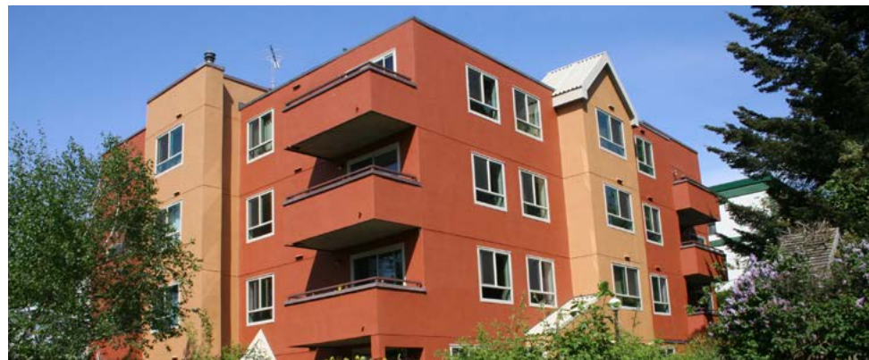
Westerdale Housing Co-operative, Vancouver
